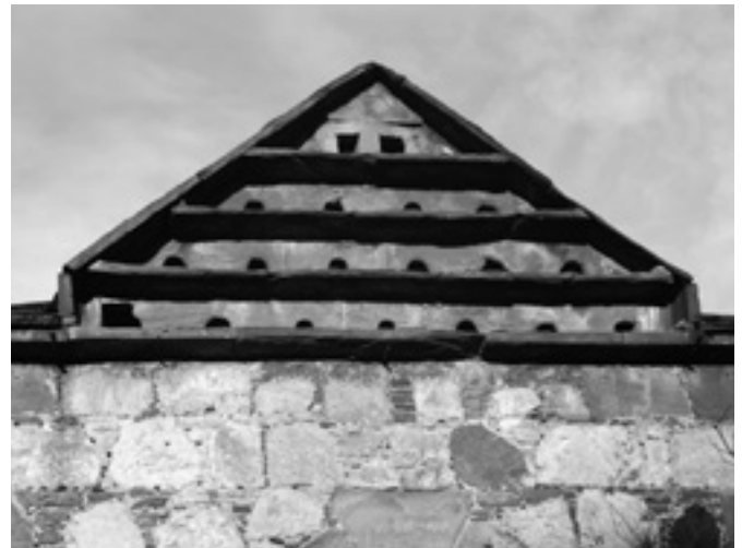
Doocot S façade with sandstone apertures to access bird roosts; facing N
