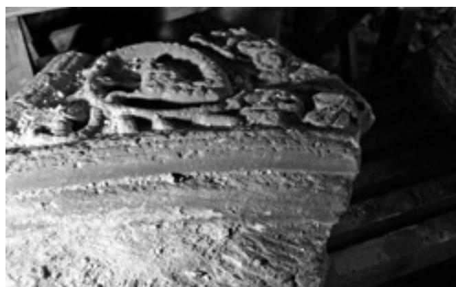
Screen spandrel detail, Kelso Abbey
