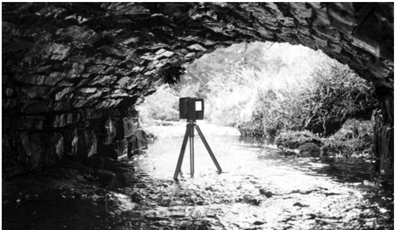
Inchnacardoch 18 th -century military bridge (measured survey) © FCS
