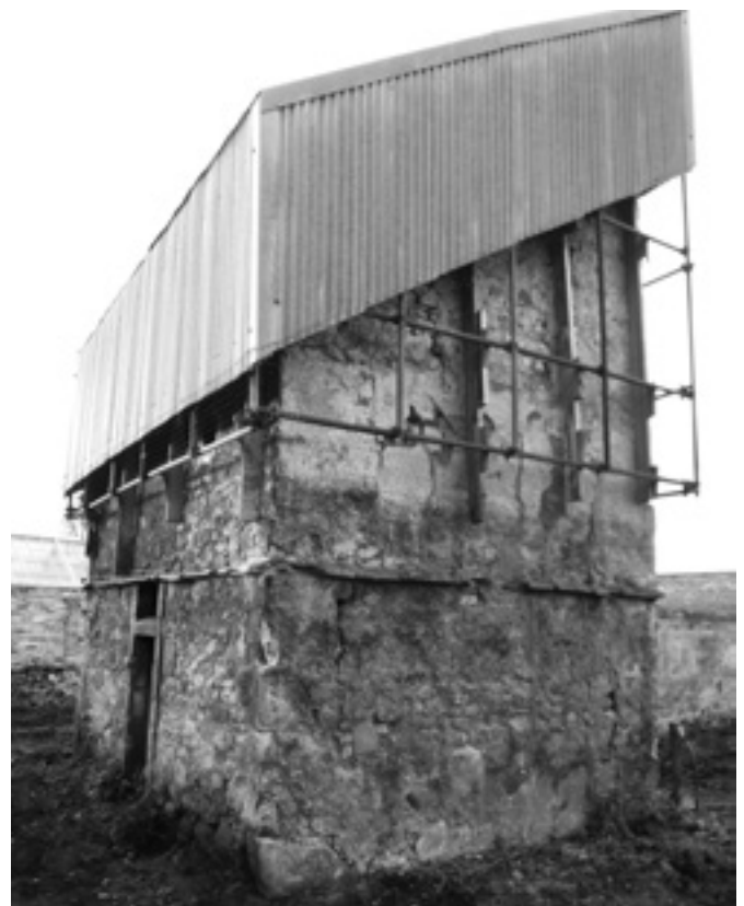
Newhailes doocot partially under scaffold, looking W
