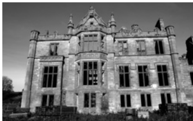
South façade Ury House west end; facing NNW
