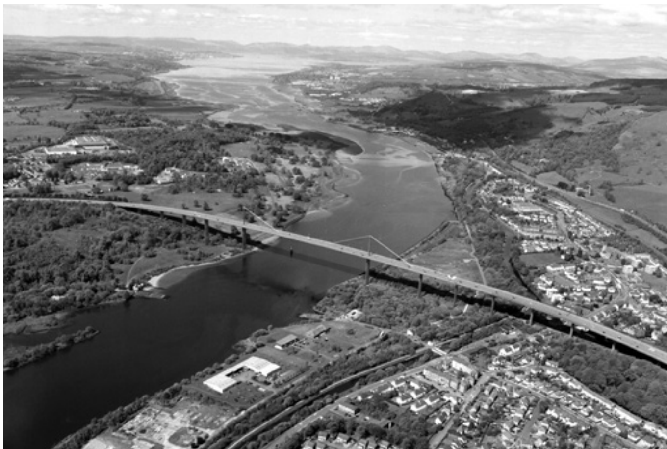
Erskine Bridge (SC 983520 Crown copyright: HES)
