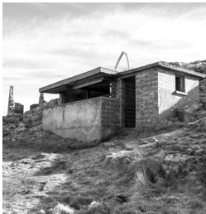
A view from the west of the military observation post built close to the summit of North Berwick Law either during or just after World War One to monitor ship movement in the River Forth. Visible above the flat concrete roof of the later observation post is a replica whalebone arch, the latest version of a structure that was first erected in the 18 th century. On the left of the image is the roofless ruin of an early 19 th -century observation post established to warn of any threat from French shipping in the Napoleonic era. (DP273592 © HES)
