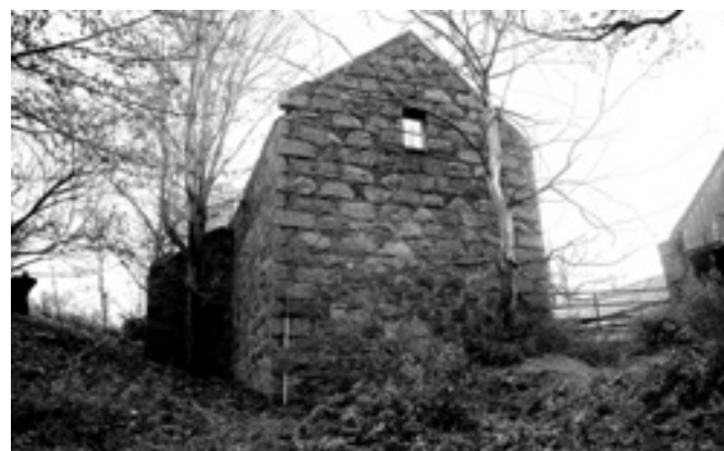
The mill at Greenhaugh
